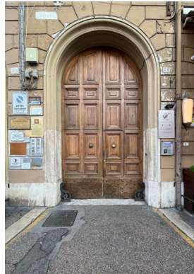
Entrance to building for the "hotel." Note lack of appropriate signage.
